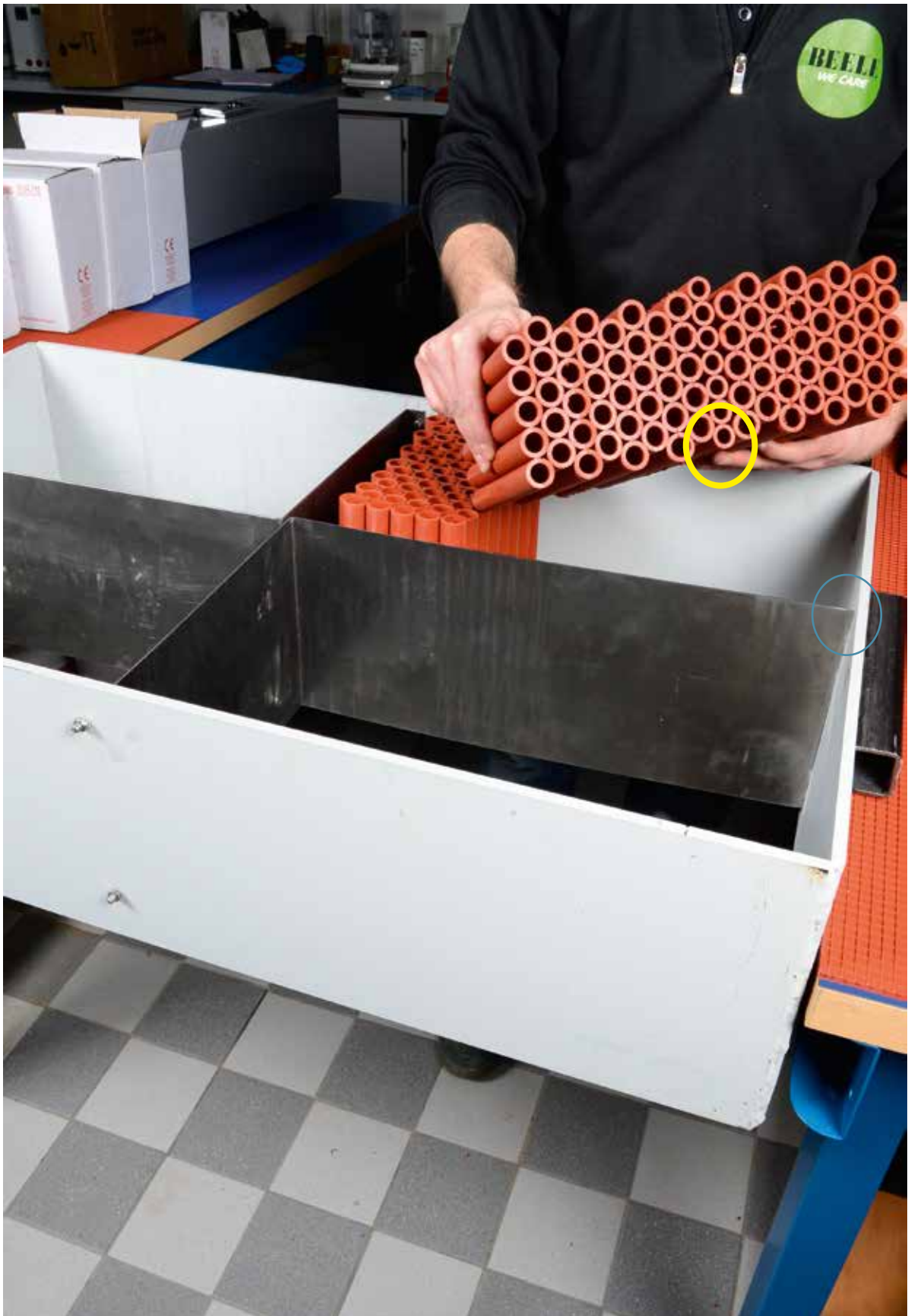
A stacked set of NOFIRNO multi-filler sleeves 22/15 with in the middle a multi-sleeve type 18/12 (yellow circle) to make the set fitting into the partition. Filler sleeves 18/12 and 27/19 are used to adjust the length of the set of sleeves. A proper fit prevents sleeves from falling down. The set with a length of ca. 300 mm is easy to handle. Note: no fixation of the steel partition at the spot of the blue circle.
