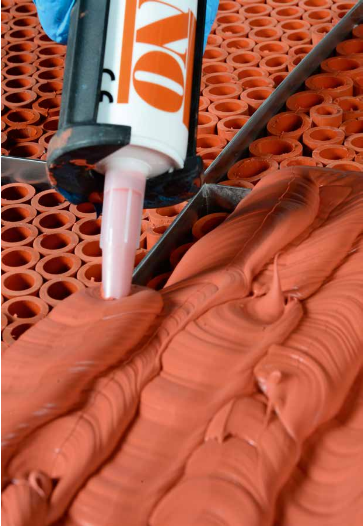
Covering the recessed steel partitions with the NOFIRNO sealant.
