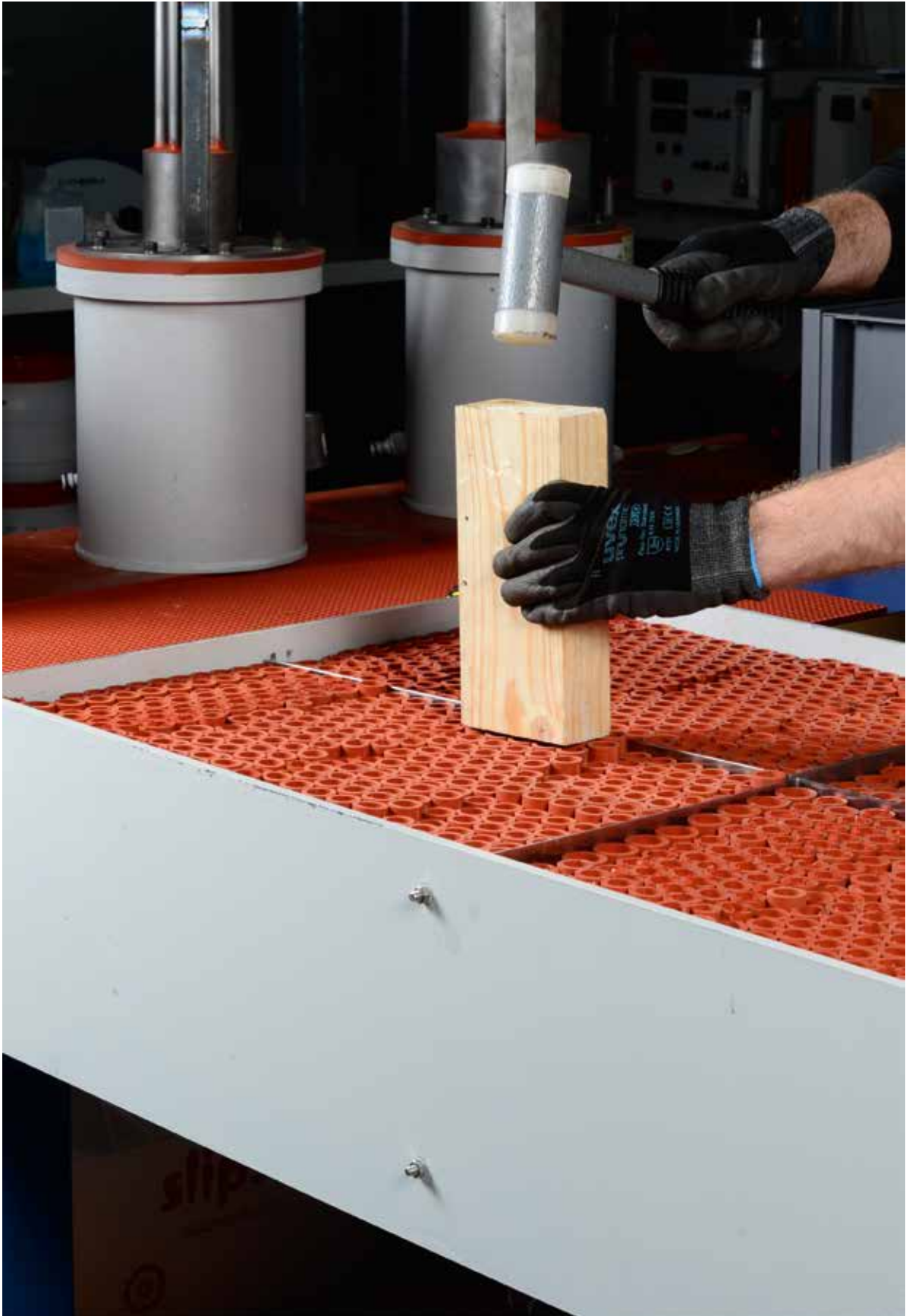
A wooden block is used to hammer the sets of filling sleeves 20 mm deep inside the sections of coaming (the gap in praxis).
