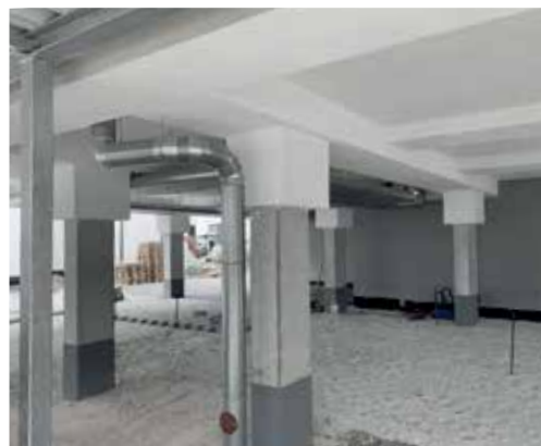
Left: Column solution implemented using Schöck Sconnex® type P.
