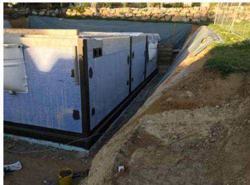
The outer strip-form sealing of the butt and construction joints is carried out with ankoX's 2C sealant SX® 1
