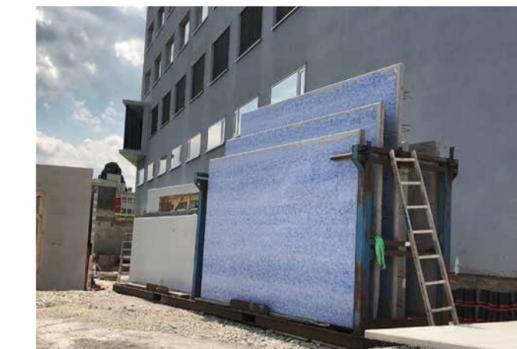
Precast wall elements integrated with Polyfleece SX® 1000 Wall delivered to the building site in a ready-to-use state
