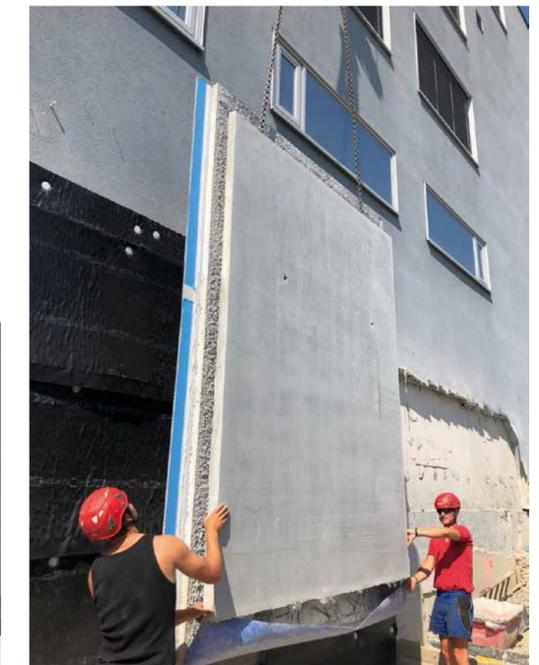
The precast concrete elements with integrated Polyfleece SX® 1000 Wall including permanent formwork allow for fast and problem-free handling on the building site
