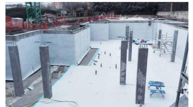
2. External, strip-form sealing of construction and crack-control joints with concrete with a high resistance to water penetration according to BRL A part 2, No. 2.53
