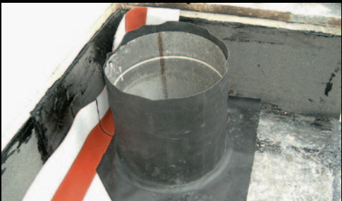
Enclosures can be vulcanized into the strip.
