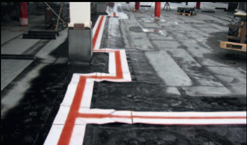
Prefabricated strips with all preforms for user-friendly fitting.
