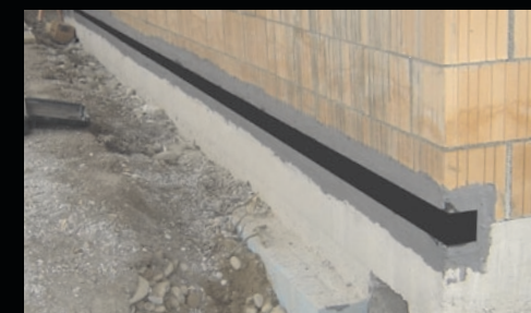
Simple and direct gluing of the expansion joint strip to walls and concrete foundations.
