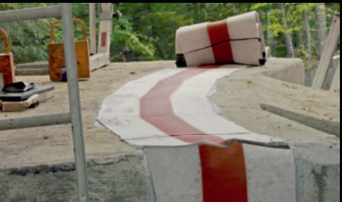
With vulcanized miter joints, the strips can be easily adapted to any changes of direction.
