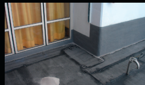
Horizontally torching into the bituminous seal and vertically glued to the substrate with epoxy resin adhesive to form a force-fit, run-free connection.
