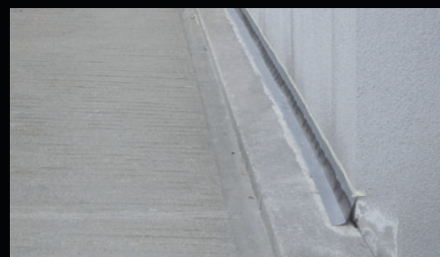
Direct gluing of the expansion joint strip to the concrete surfaces.
