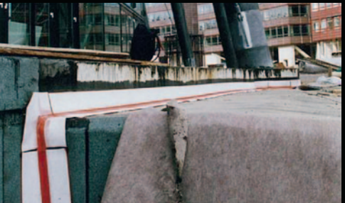
Safe sealing of building transitions between old and new buildings.
