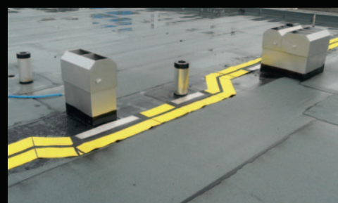
Special plate transition and interim pieces for connection to metal work.
