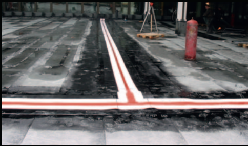
Combination of various strip types (e.g., transitions RL 100-40).
