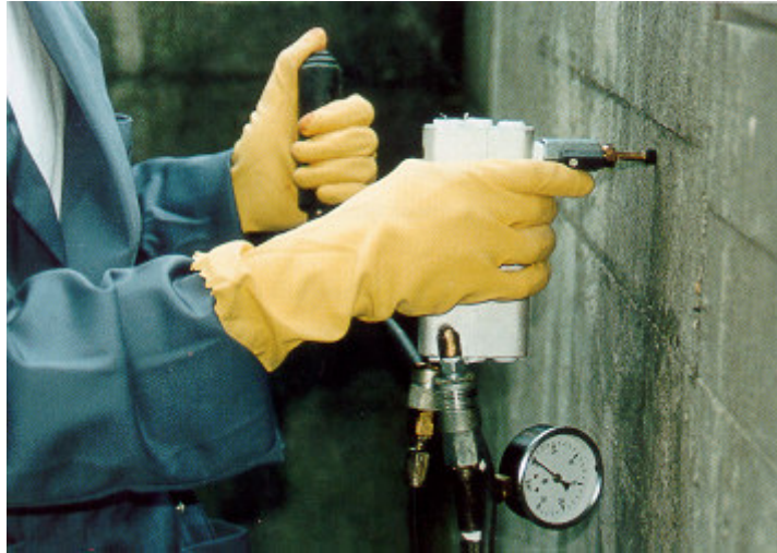
Photo: Injection with epoxy resin
