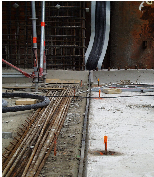
Photo: Injection tubes (orange) sticking out of floor
