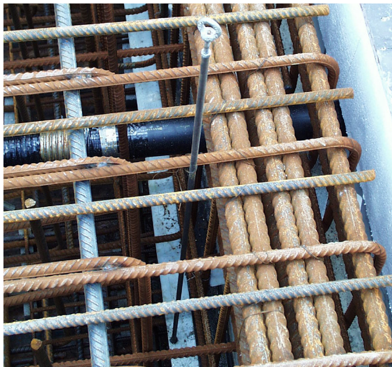
Photo: installed injection system before pouring
