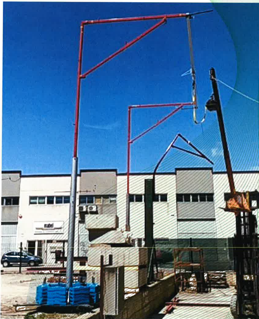
Fig. 4: Anchor device type D (type Horizontal SafeAccess and NAV2 trolley made by FALLPROTEC SA) with anchors of type AluPercha and mobile base units
